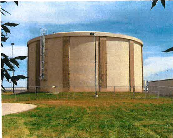
ABOVE: DePere, WI, 3.0 MG water storage tank. Fluted, concrete pilasters effectively break up the exterior appearance to help this tank blend with local surroundings.
