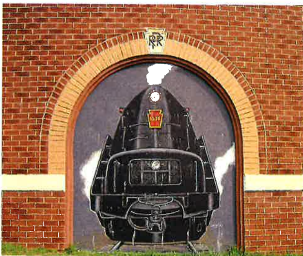
ABOVE: Altoona, PA, 5.7 MG water storage tank. The brick face facade replicates the locally historic railroad roadhouses. The treatment links the tank to Altoona's past, reminding passersby that the City's original reservoirs were constructed by the Pennsylvania Railroad.
