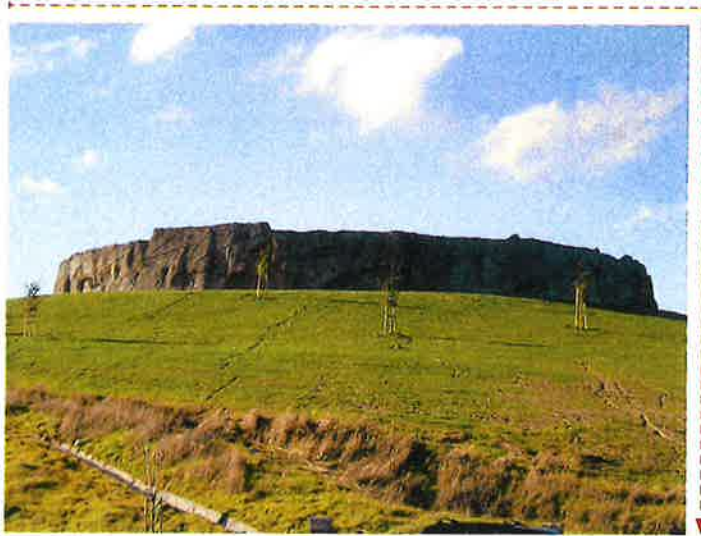
RIGHT: Brentwood, CA, 4.0 MG water storage tank. The architectural rock facade make this partially buried tank look as if it's been a natural part of the topography since the Ice Age!
