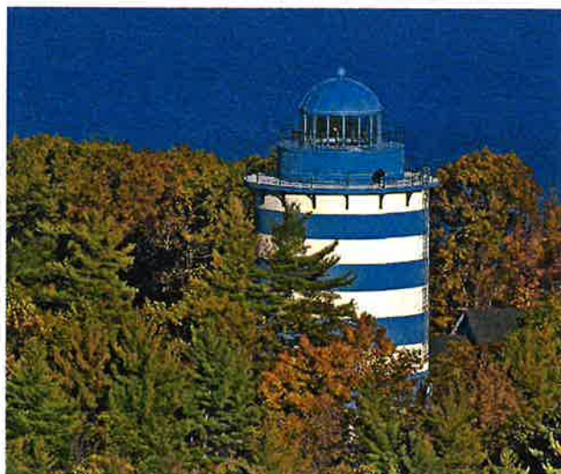
ABOVE: Laconia, NH, 500,000 gallon water storage tank. A landmark is created for a major development overlooking New Hampshire's Lake Winnepesaukee by transforming the water storage tank into a lighthouse.
