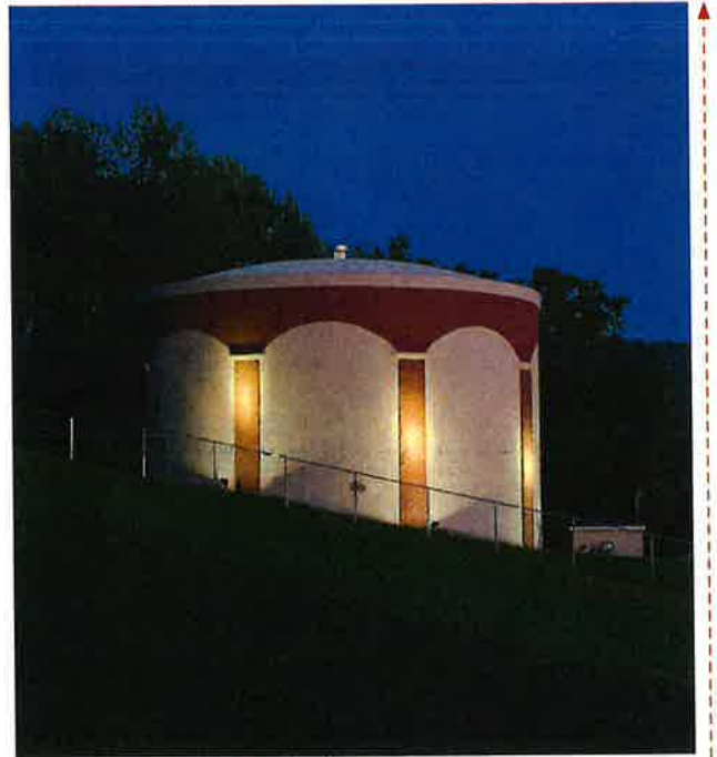
ABOVE: Vestal, NY, 1.0 MG water storage tank. Simulated EIFS arches combined with brick pilasters give this tank a stately appearance while the lighting provides both security and elegance.
